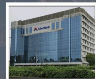
Allied Bank Limited, Head Office Lahore
